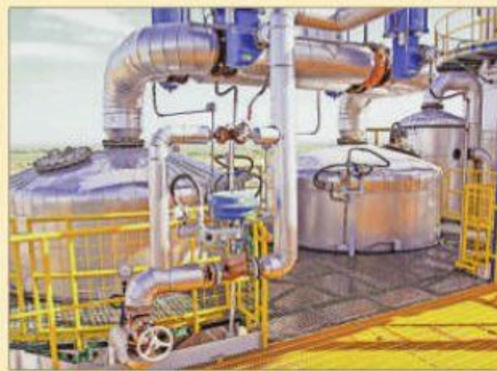
■ Deficient monsoon in Maharashtra, Karnataka could lower sugarcane output in 2026-27
