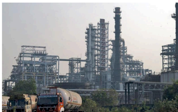
STILL WORKING. The constraint comes as Indian Oil enters the final phase of its ₹17,825-crore Petrochemicals and Lube Integration Project. The expansion started five years ago BLOOMBERG
