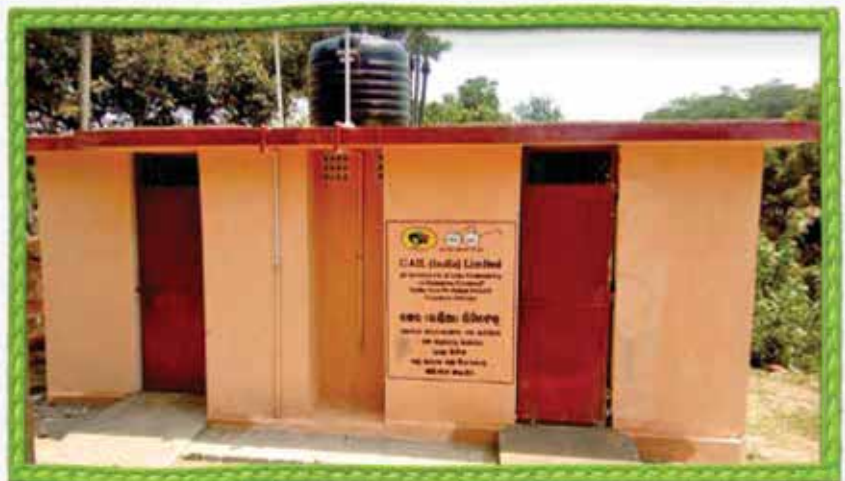
Construction of Toilet under Swach Bharat Swach Vidyalaya
