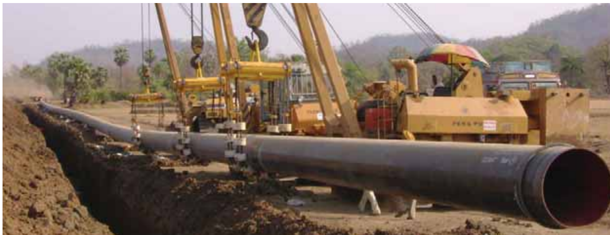
Pipeline Laying Operation
