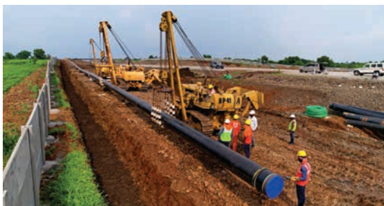
Laying of Natural Gas pipeline from Mumbai to Nagpur under MNJPL project
