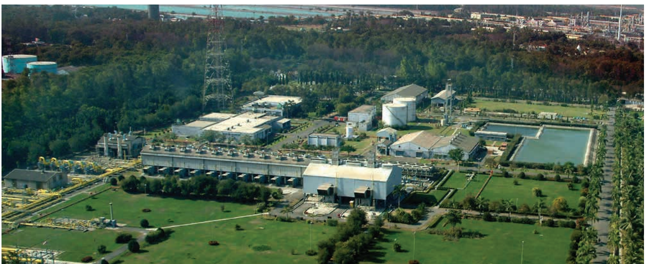
Aerial View of GAIL, Hazira
