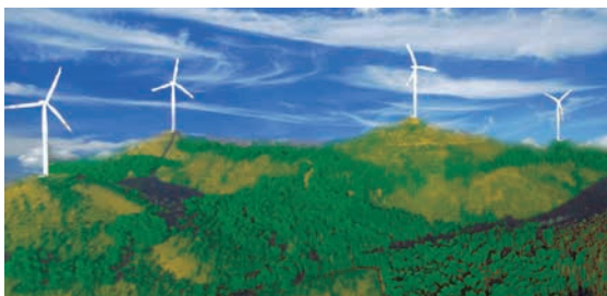
Wind Energy assets of GAIL in Hassan, Karnataka
