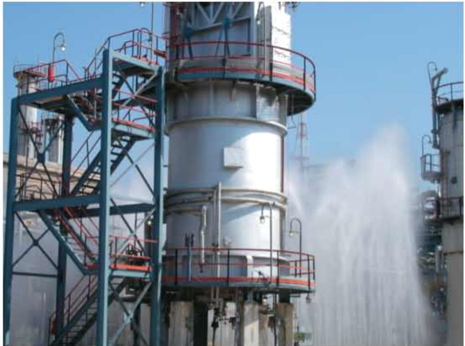
Water Curtain Development during Fire & Safety drill - Pata, U.P.
