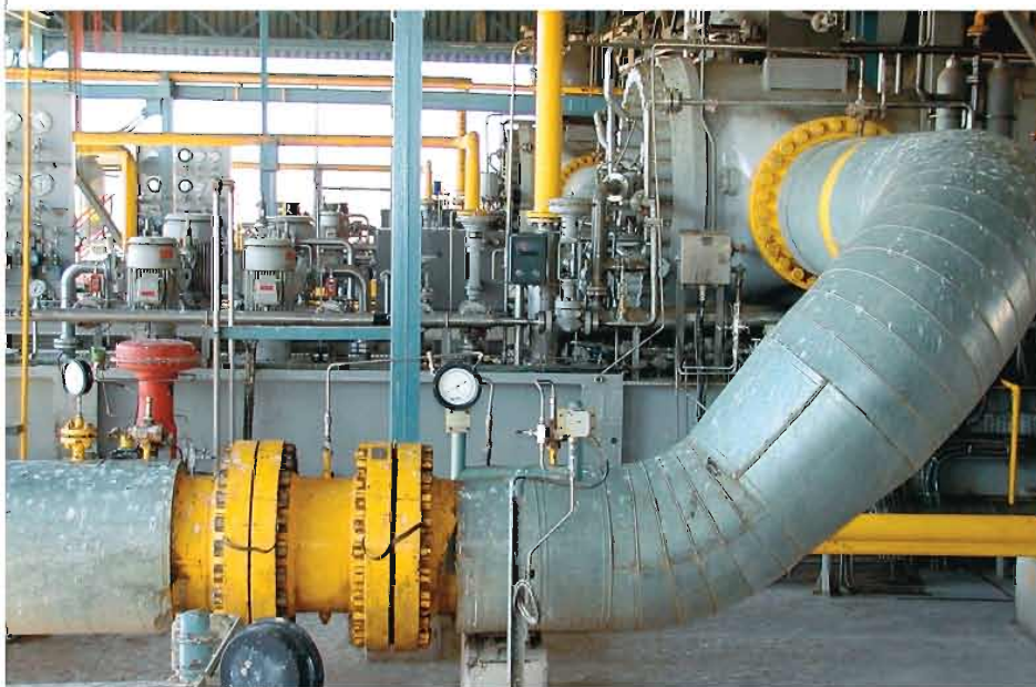
Gas Turbine at GAIL, Vijapur, M.P.
