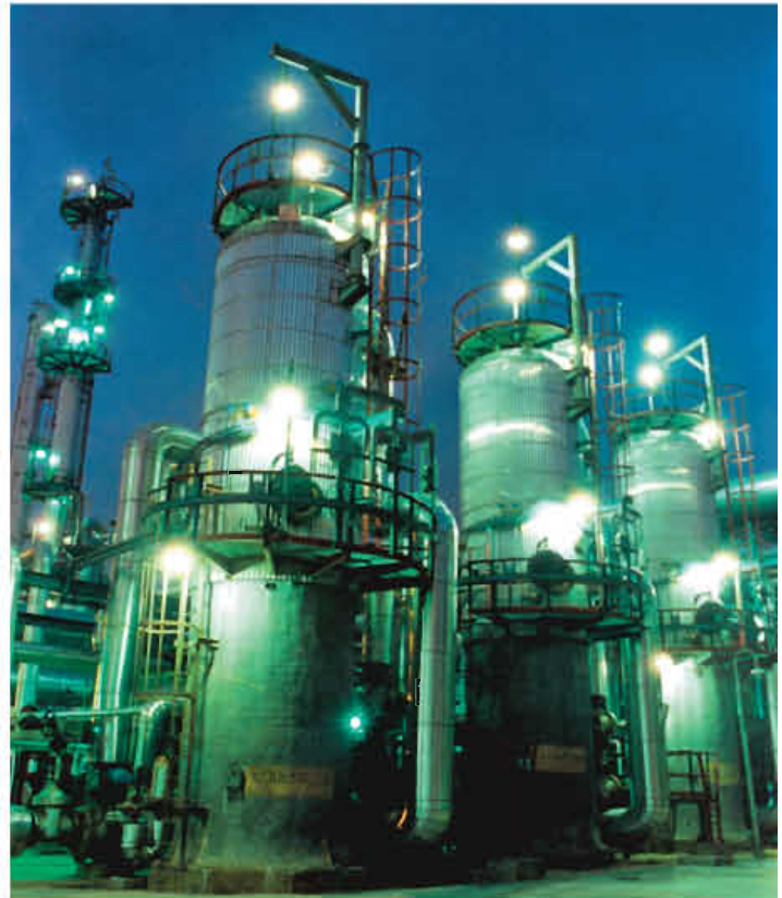
Night shot of Pata Petrochemical Complex showing the cold section column of Gas Cracker
